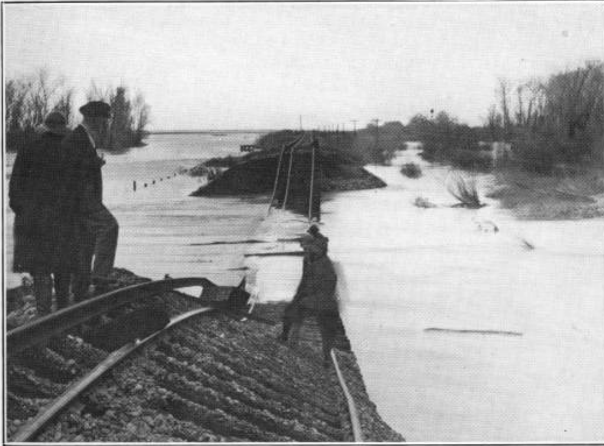
Break in east levee of the Feather River just south of Marysville during flood of January, 1914.
